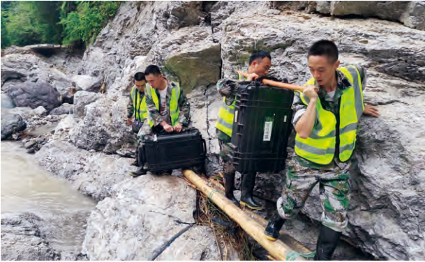
■ Our workers at Meishan subsidiary hiked 10 kilometers carrying 100 kg of equipment to repair the communications network
