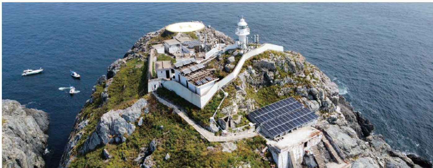
China Mobile's Zhoushan Zero Carbon Base Station
