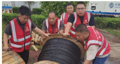
Maintenance staff carried out optical cable repairs
